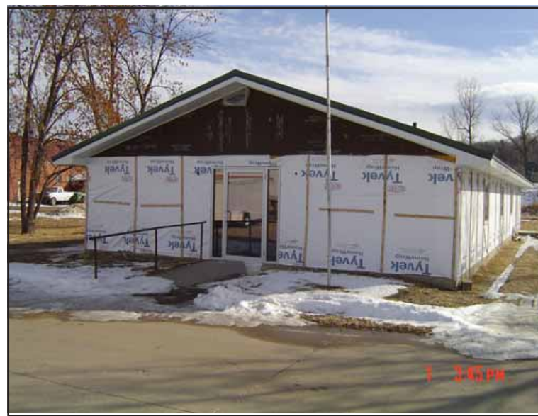
New doors were recently installed on the Senior Center
