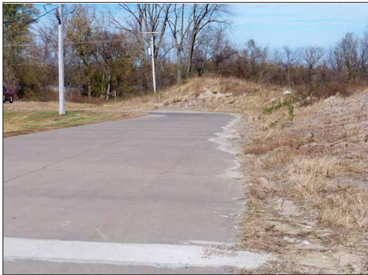
Existing levee from Highway 92 North to the railroad tracks
