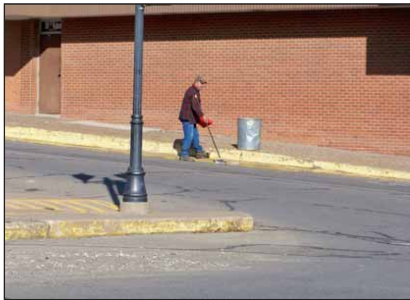
Clean up work on the Columbus Junction State Bank sidewalk
