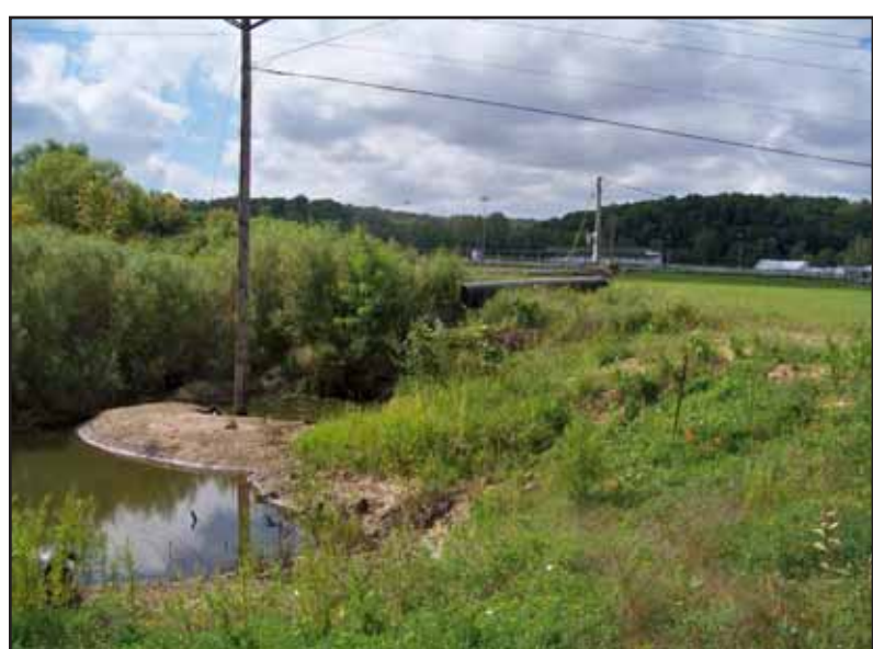
New culvert being installed at Fairgrounds
