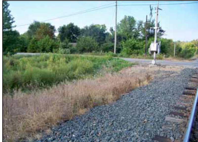
Culvert on Highway through Fredonia
