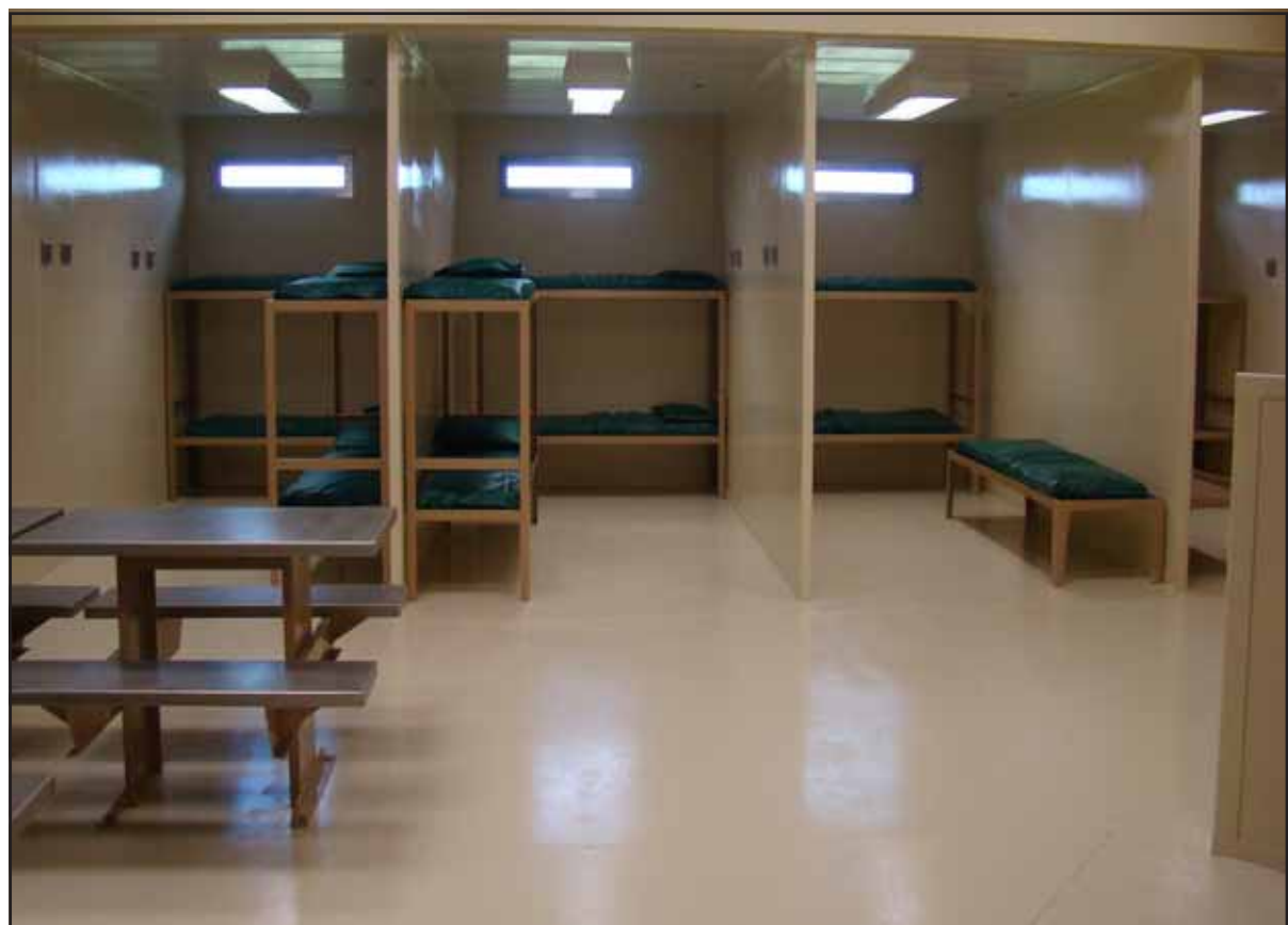
The men's dormitory in the new Louisa County Jail provides 14 beds. Costs were reduced by eliminating the need for additional doors, plumbing and security electronics. There are two-inch thick concrete walls between bed areas, instead of traditional concrete blocks, provides more space for beds as well as savings on heat and air-conditioning. Submitted by Connie Street.
