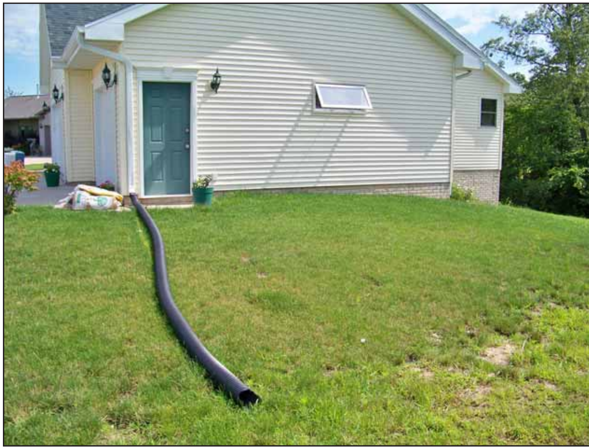
Proper way to drain downspouts away from your home.
