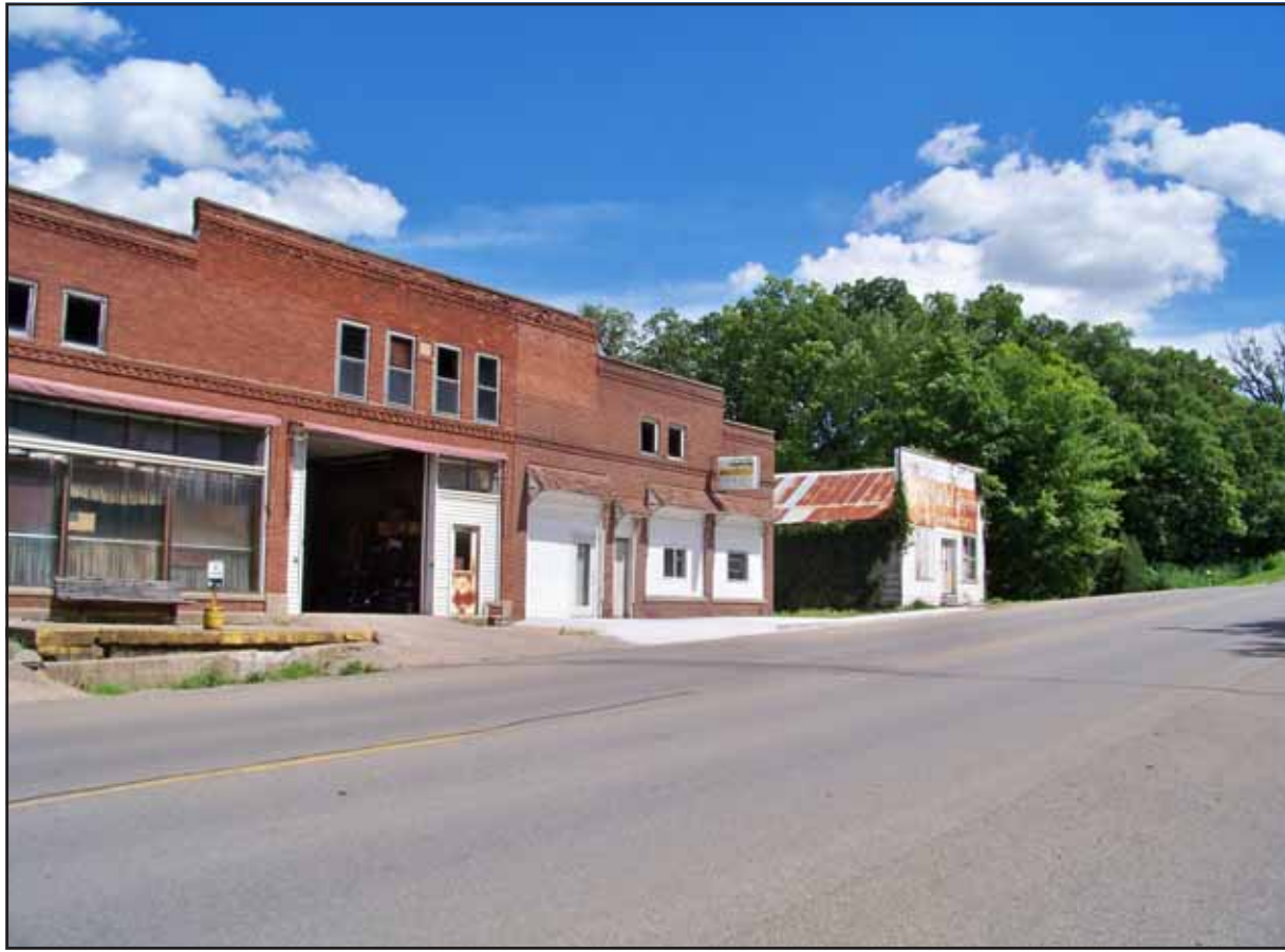
Area on Main Street proposed for combination auto parts store and bar
